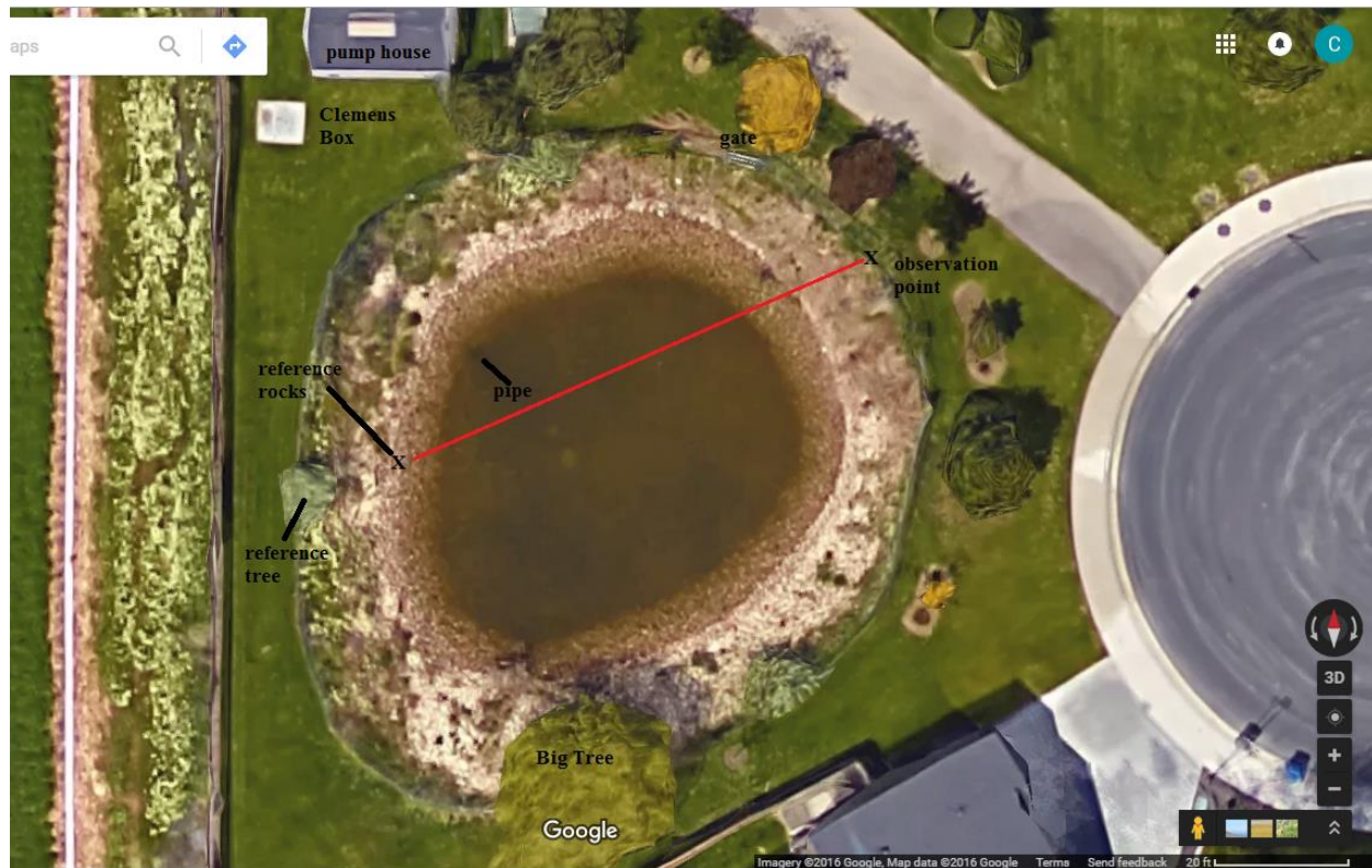
Figure 8. Observation and reference points for measuring drop in pond water level by the ruler gauge method. Also shown is the location of the pipe from the pond to the Clemens box.
